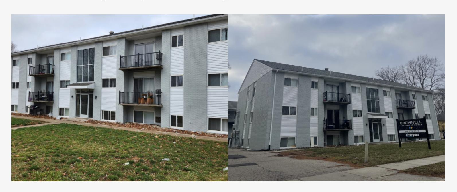
The two pictures above show the building after the paint job was complete as well as all 4 balcony railings replaced with 36 inch high, black aluminum rails.
